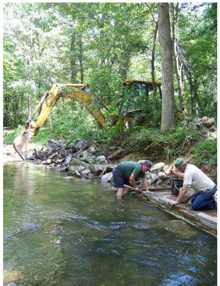
Below: Attaching boards to the log
